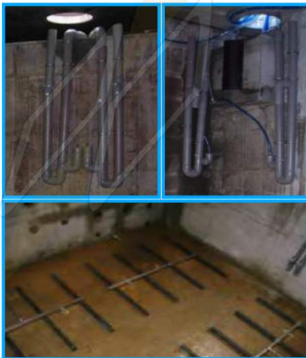
INSIDE VIEW OF TANK
